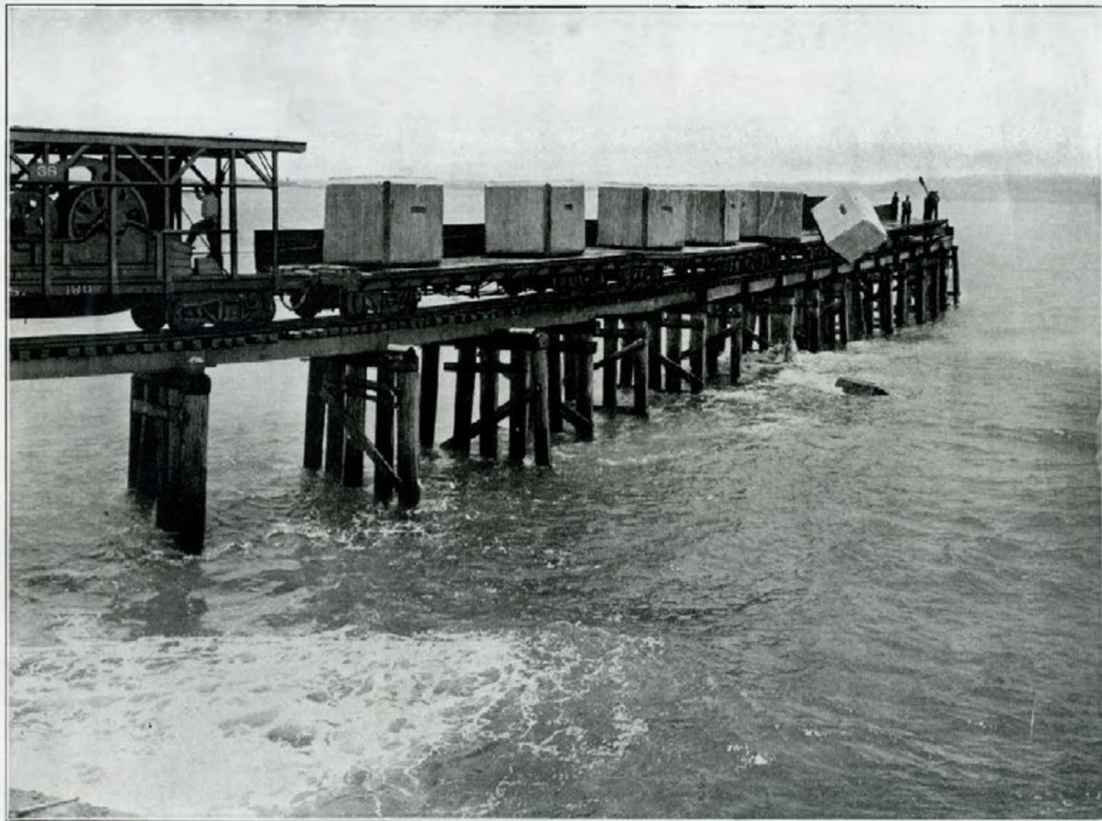
Dropping 25 ton Concrete Blocks into Limon Bay. These blocks form the Foundation of the Breakwater, Panama Canal.
